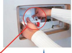
maximun length. - Press the holder that fixes the lever block to remove it.
